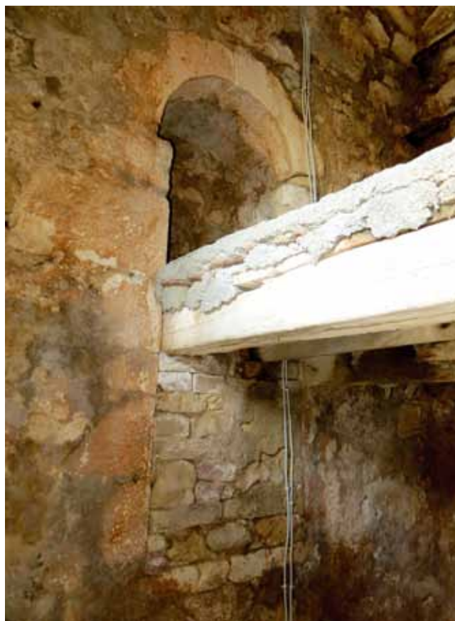
4. Zazidana monofora istočne stranice trećeg kata zvonika (foto: E. Motušić) Walled-up single-light window on the east side of the third floor of the bell tower
